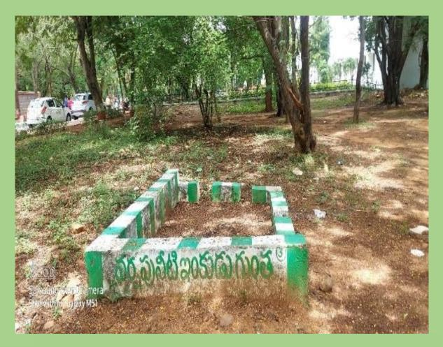
Fig: Rain water Harvesting Pit
