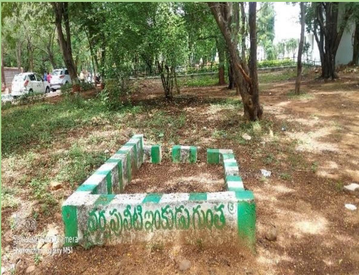
**Fig: Rain water Harvesting Pit**
