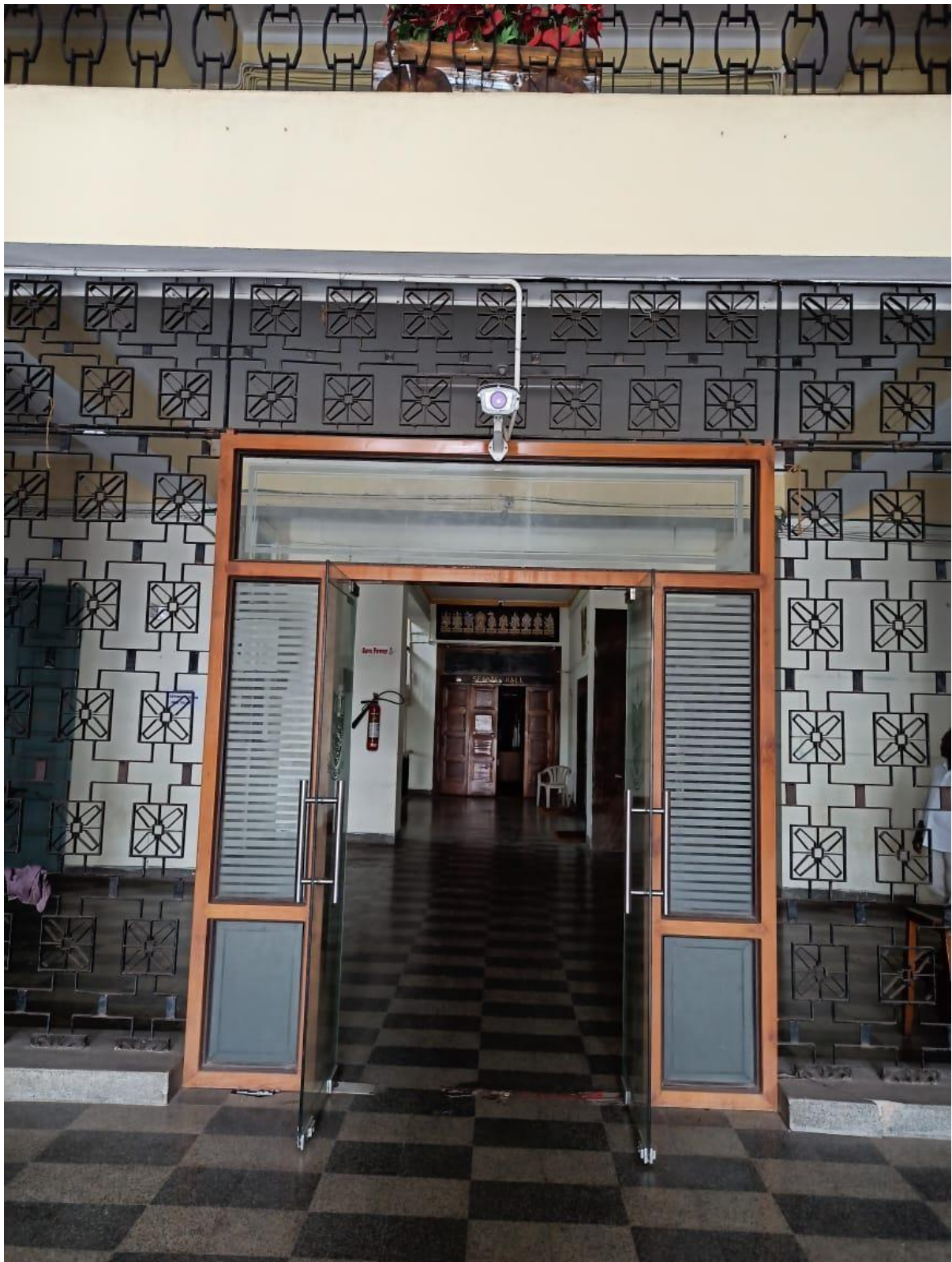
Installation of CCTV Cameras Throughout The Campus
