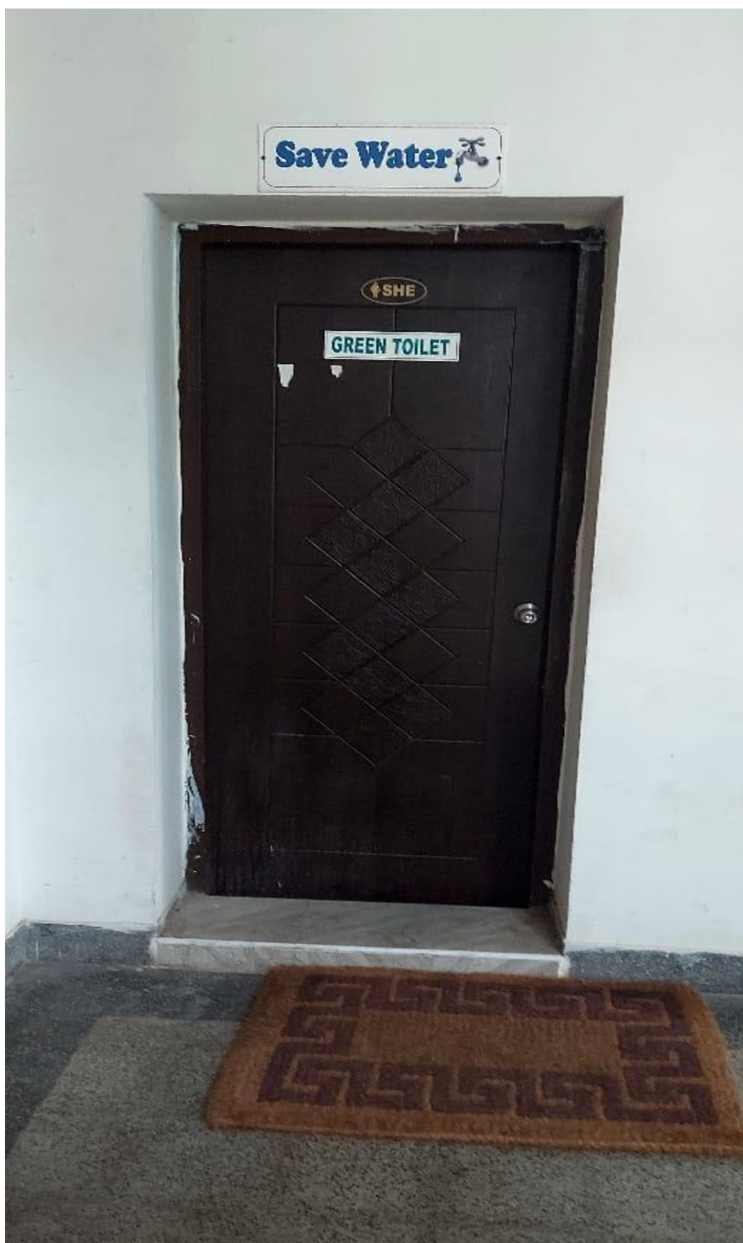
Green Toilet Facility for Women
