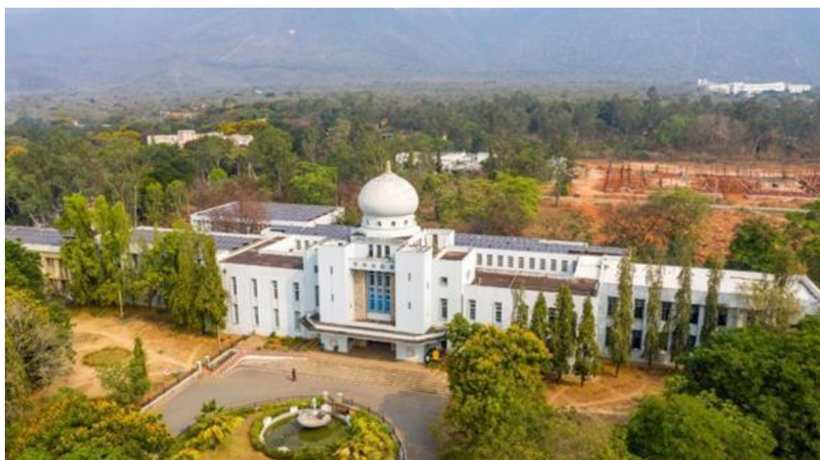
Solar Panel at SVU Library
