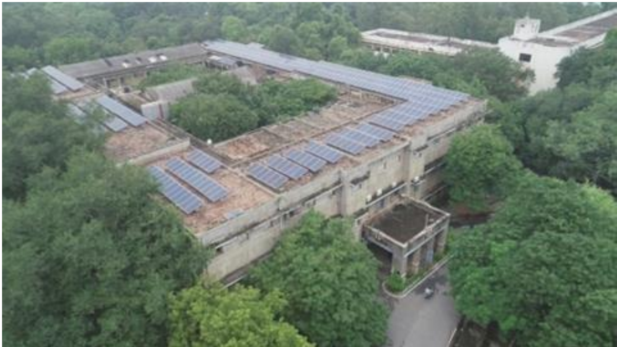
Solar Panel at Prakasam Bhavan
