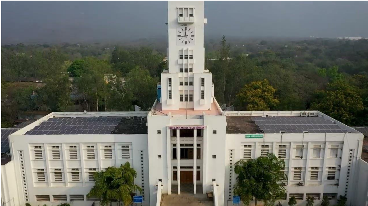
Solar Panel at SVU Administrative Building
