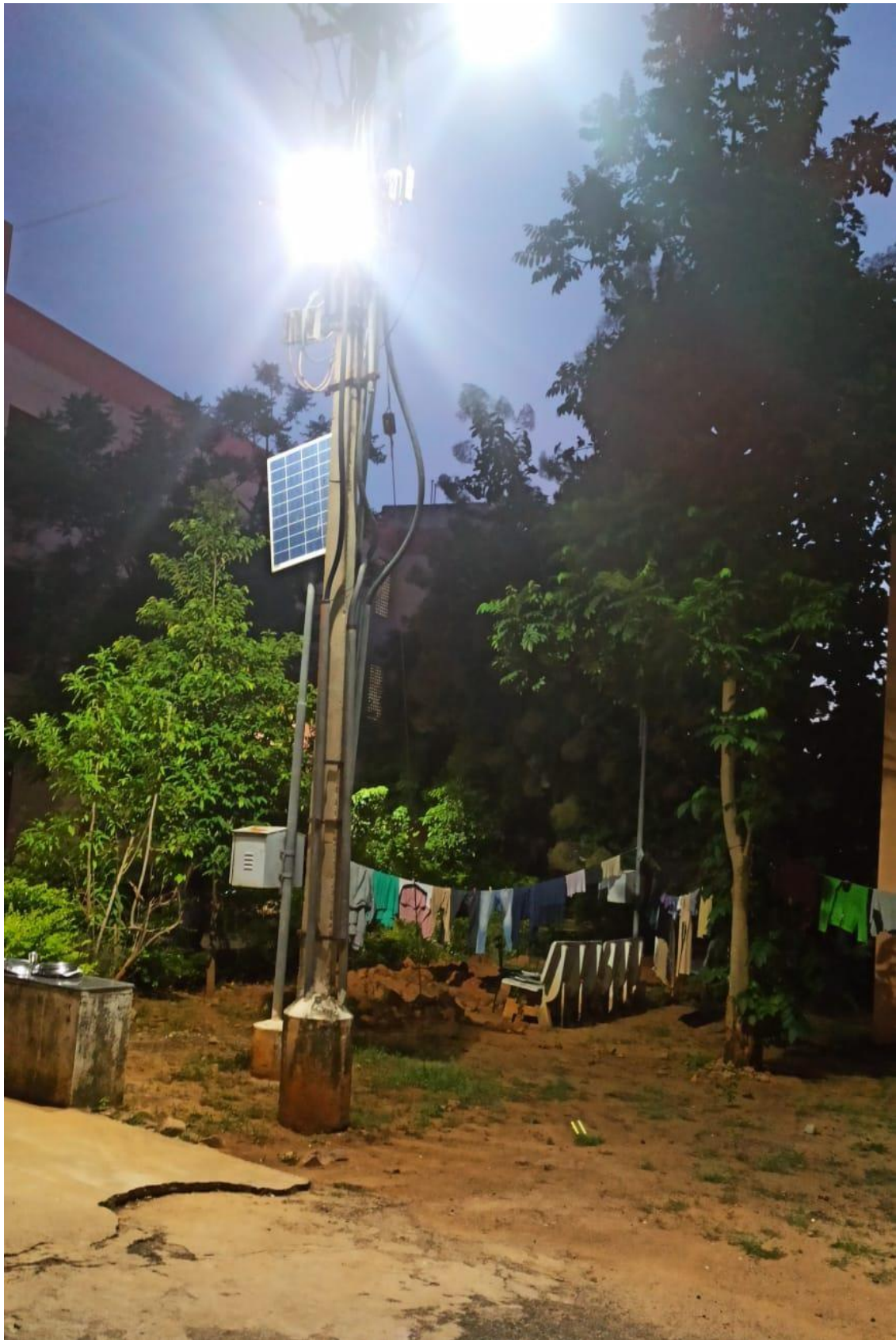
Solar Panels are exported to the Grid of Electricity
