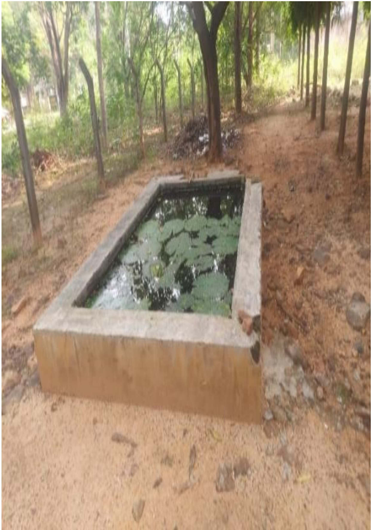
Rain Water Harvesting
